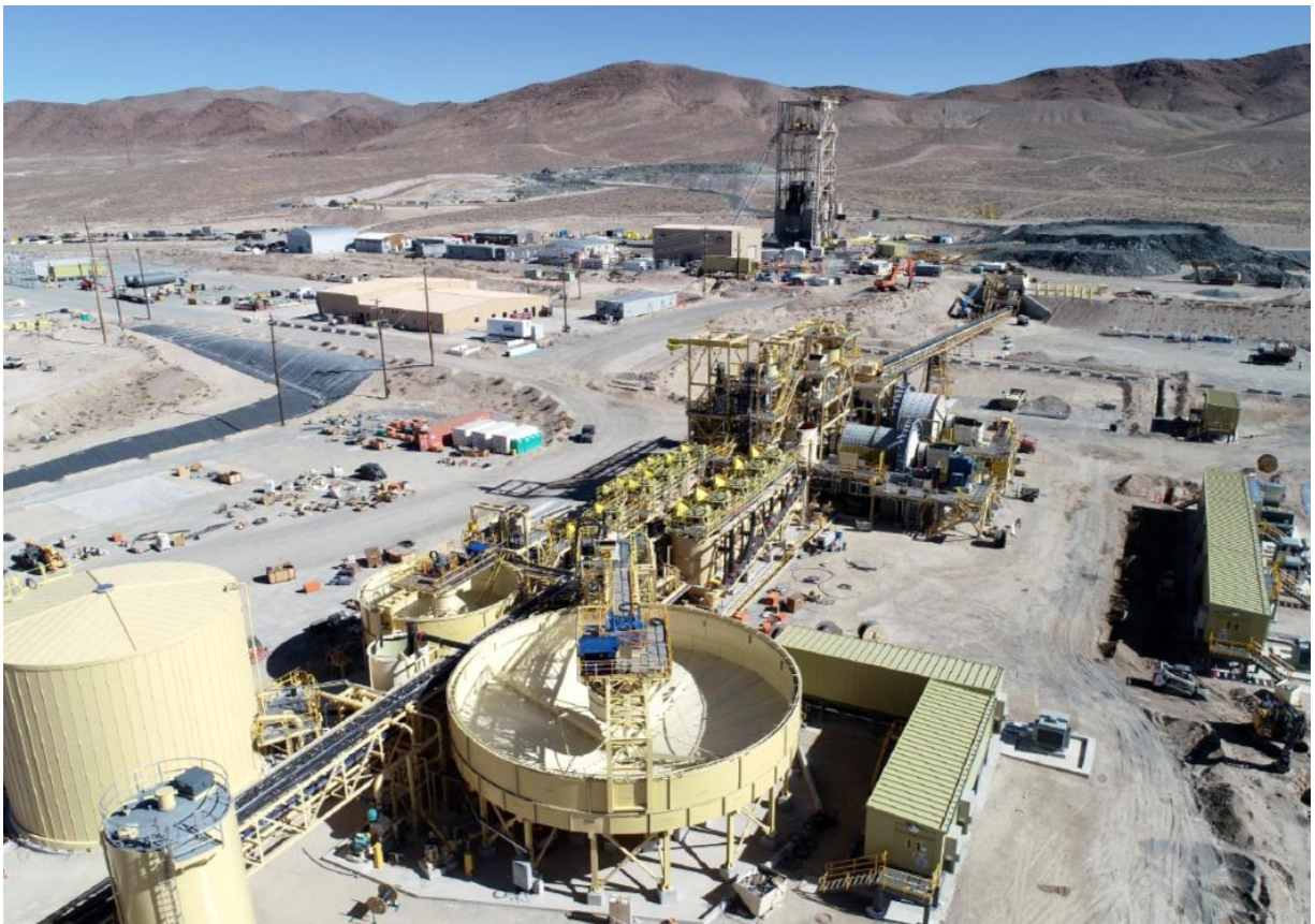
(Process plant, admin building and main headframe looking east)
