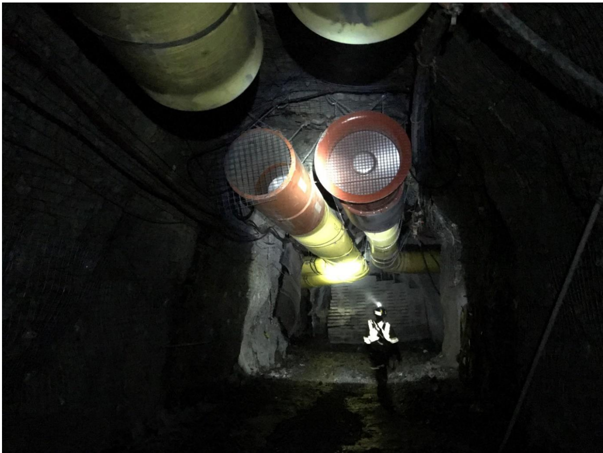
(Ventilation upgrade on the 2850 level)
