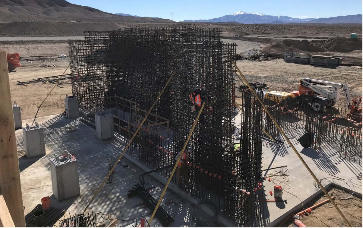
(Sag Mill foundation)
