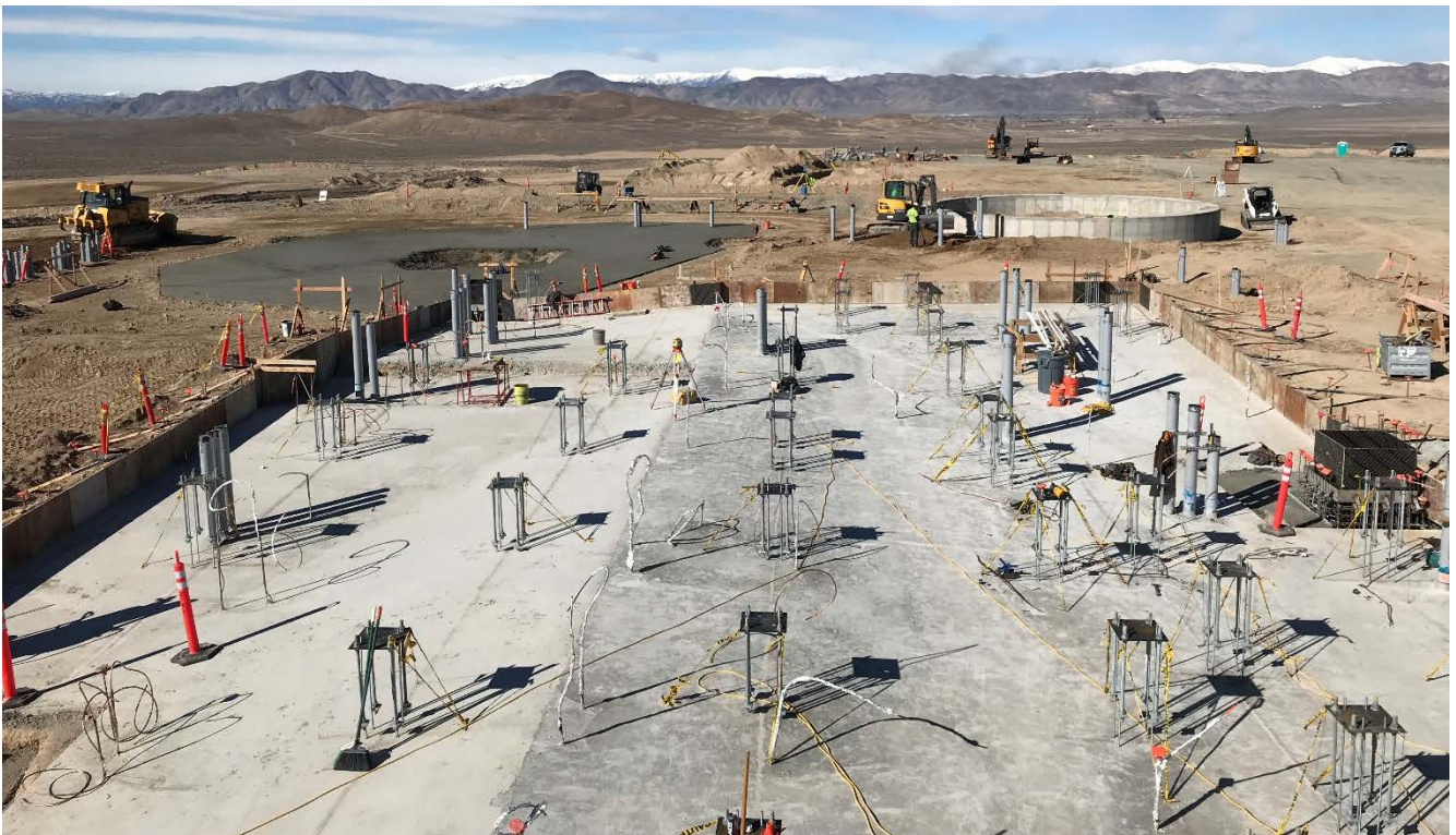
(flotation deck foundation)
