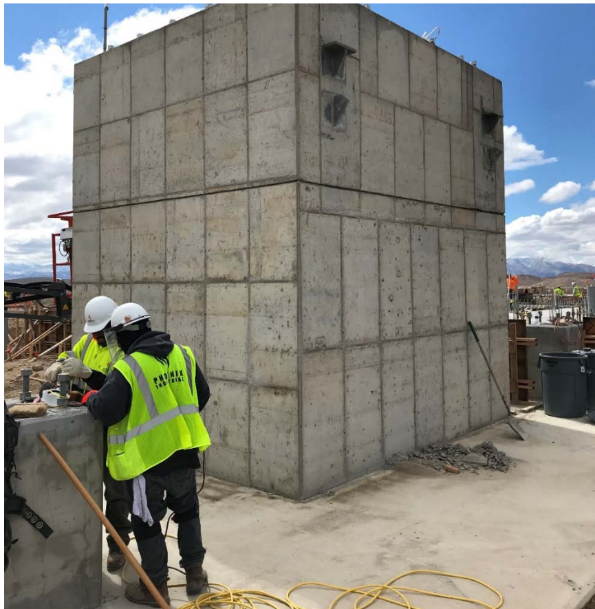
(Completed concrete for the vertical mill)
