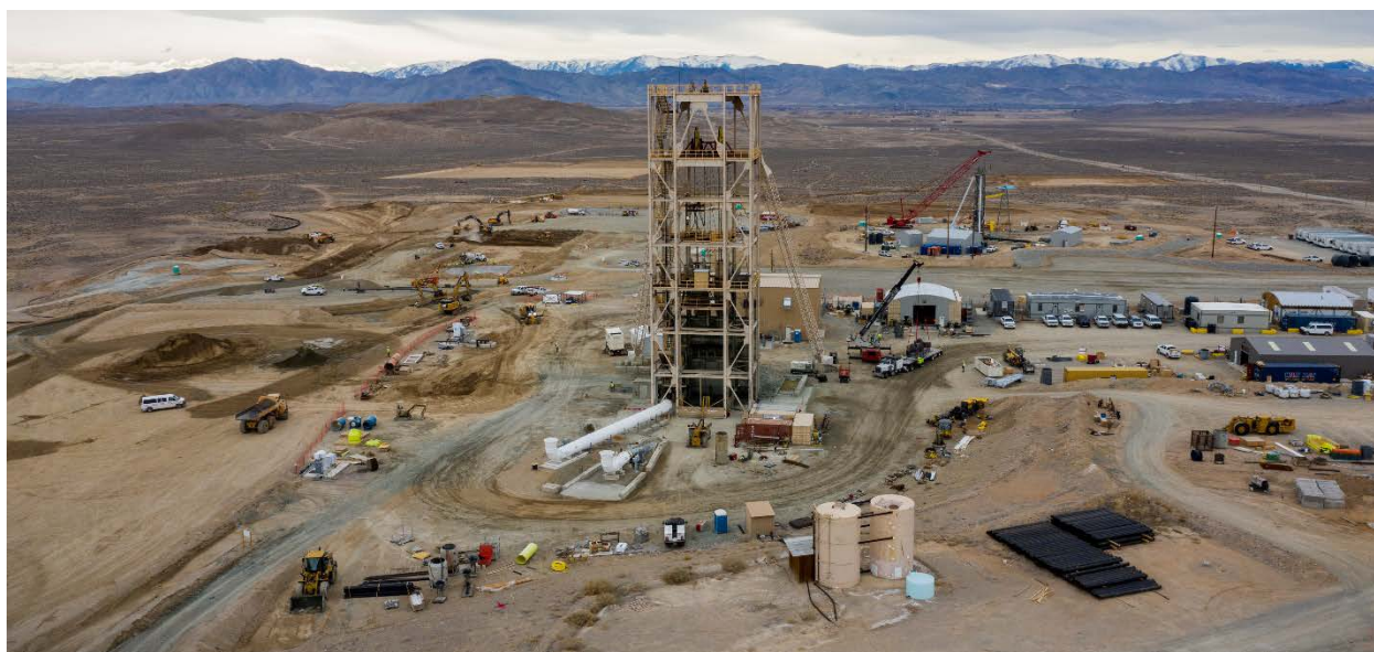
(Main shaft headframe, east north vent shaft headframe and surrounding works)
